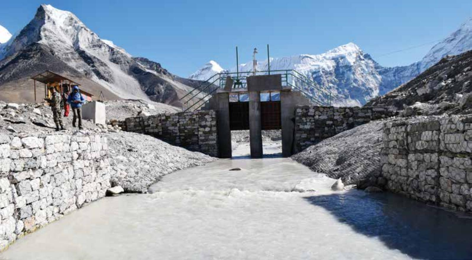
The construction of an artificial open channel helped lower the water level in Imja Lake by 3.4 metres.
