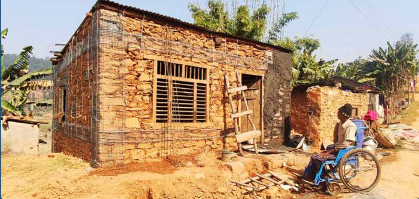
HOUSE BEING RETROFITTED IN GORKHA.
