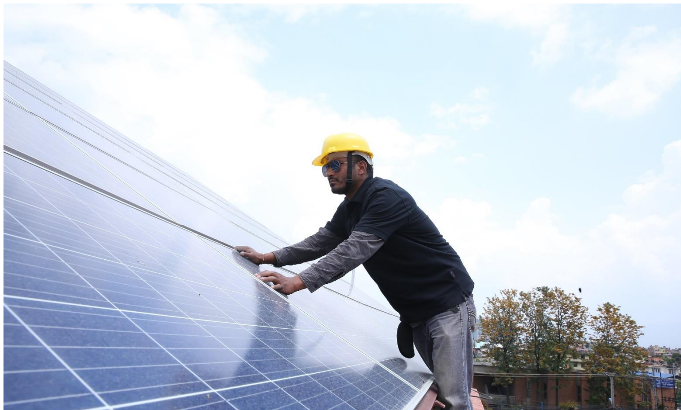
Figure 23: A worker fitting solar panels. Photo credit: UNDP Nepal
